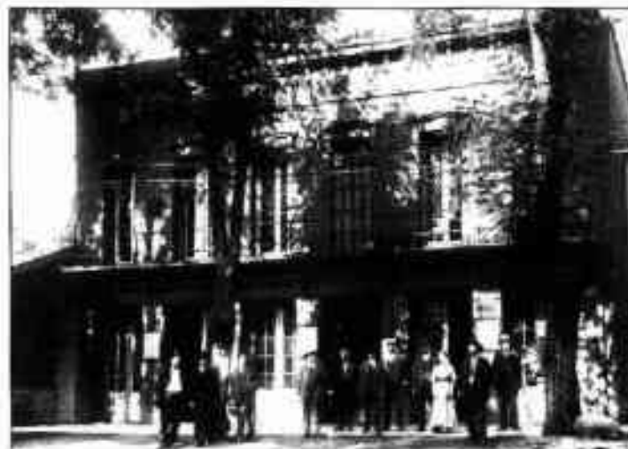
Many cow county courthouses survive from gold rush days. This one in Weaverville, constructed in 1857, first housed The Apollo Saloon, the county's first piano, and a business of ill-repute.
